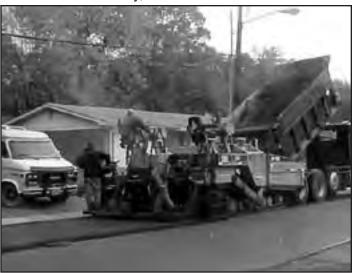
Sherrell Construction Company working to put asphalt overlay on Forest Home Drive.
