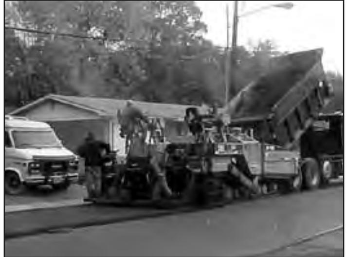
Sherrell Construction Company working to put asphalt overlay on Forest Home Drive.
