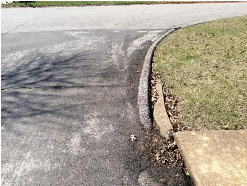
Existing Asphalt Curb Typical Example
