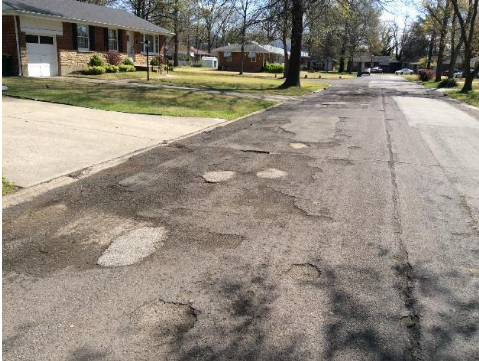
'2' Rating – Mead Drive – Overlay – Severe Potholing & Raveling
