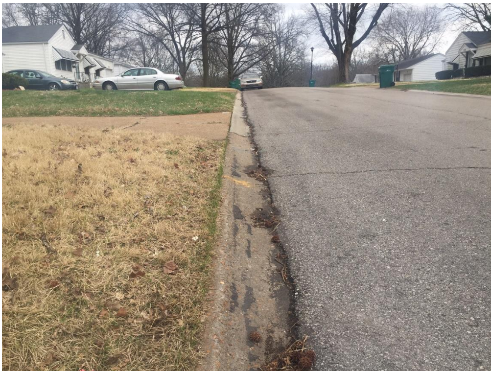
Example - Lack of Waterproofing Edge Sealant
