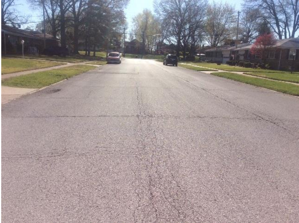
'5' Rating – Crete Drive – Overlay – Moderate Reflective & Block Cracking
