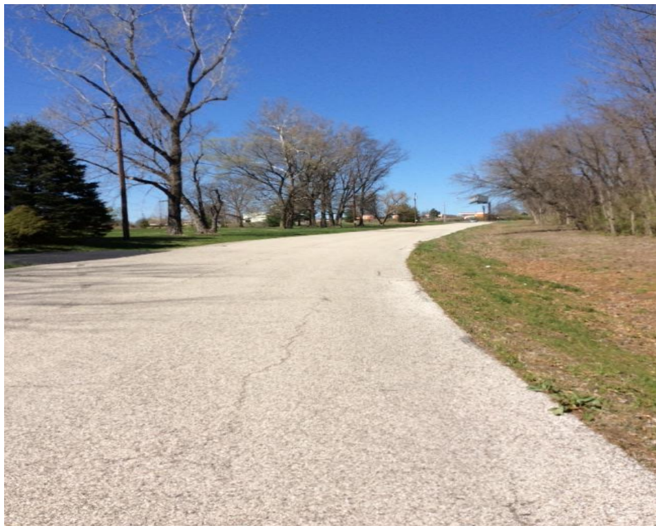
'6' Rating – Raftery Lane – Full Depth Asphalt – Minor Cracking
