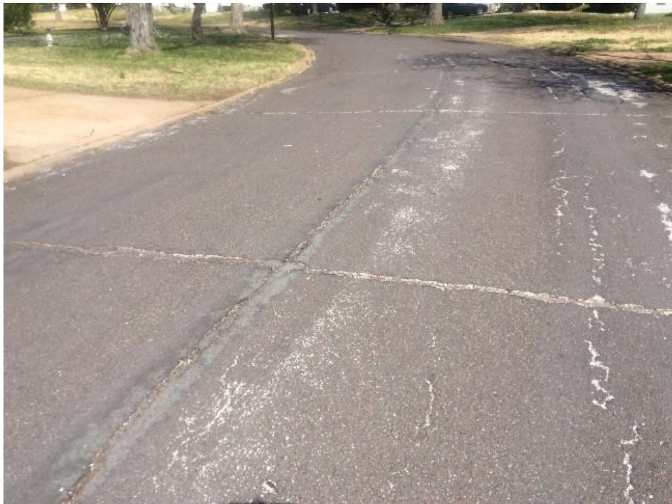
'4' Rating – Fathom Drive – Overlay – Significant Reflective Cracking
