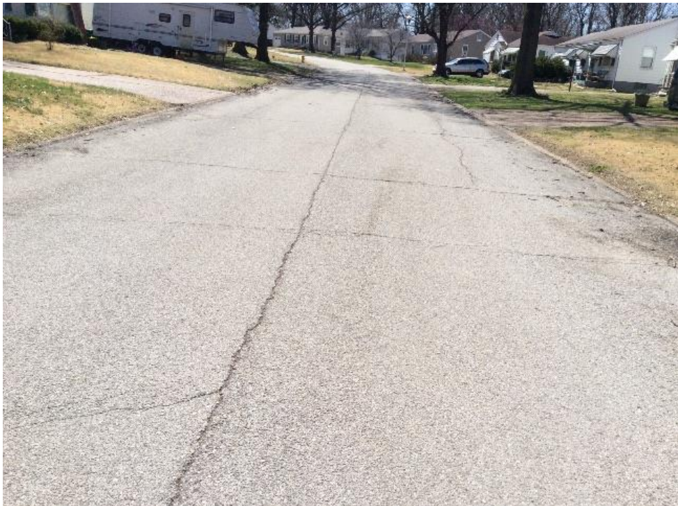
'2' Rating – Toelle Lane – Full Depth Asphalt – Severe Block Cracking
