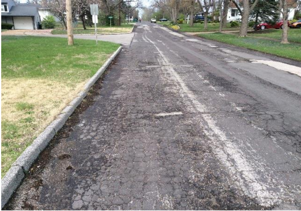
'2' Rating – Toelle Lane – Full Depth Asphalt – Severe Block Cracking
